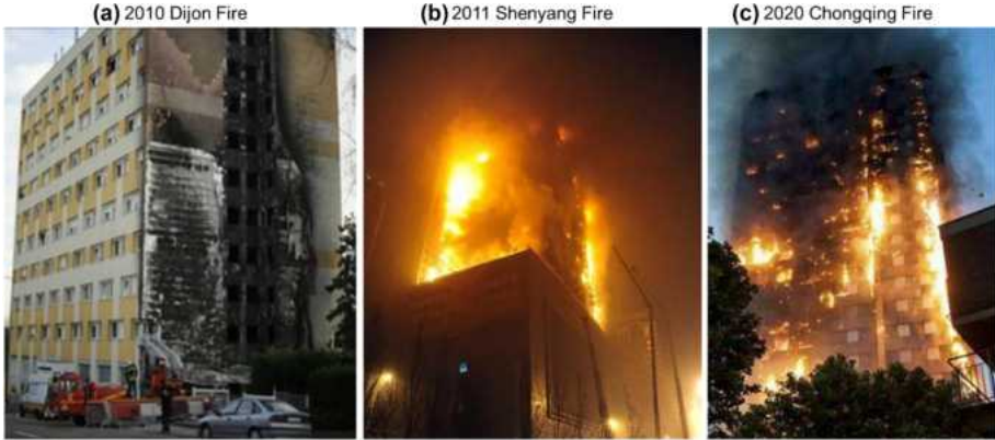
Figure 1. Typical EPS ETICS facade accidents, a Dijon fire, France in 2010 https://www.bbc.com/news/world-europe-11752303 , b Shenyang fire, China in 2011 http://news.sina.com.cn/c/2011-02-08/153321924087.shtml , and c Chongqing fire, China in 2020 http://cmszfb.oss-cn-beijing.aliyuncs.com/u/cms/www/202001/02143433gso9.jpg .
